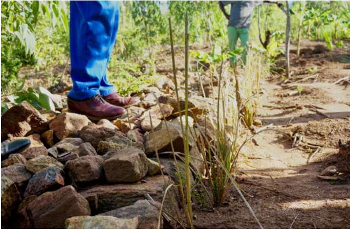
Field site visit to see restoration practices. The barrier of rock and grass help slow the water flow and allow plants to grow. (Source: Flickr)
